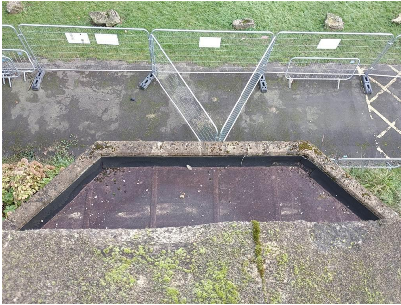
Left: existing felt to one of the window bays
