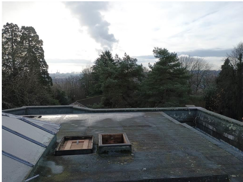
Above: main flat roof (felt)
