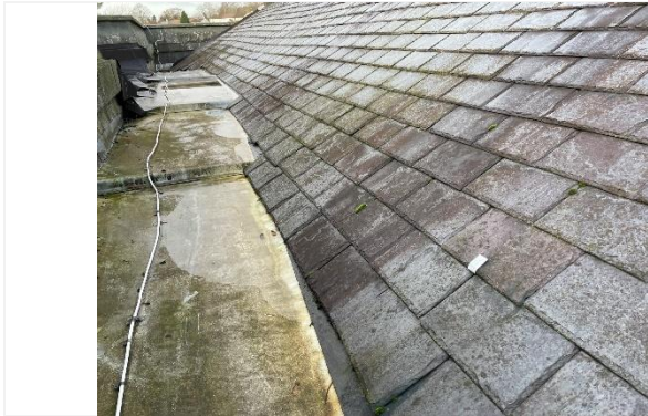
At the pitched roof abutment, the bottom two or three courses of tiles will need to be removed and safely set aside. This is to allow for the new system to be installed correctly.
