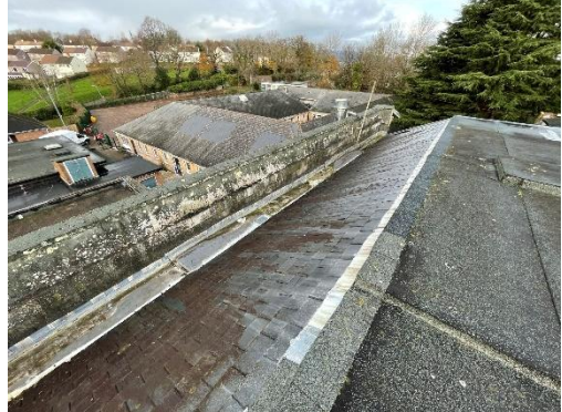
General overview of existing roof area, opposite side.
