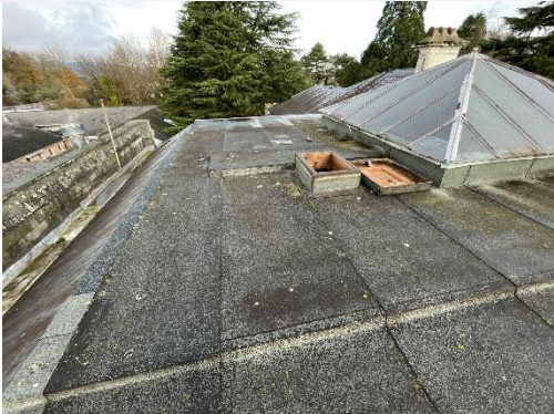
Overview of Roof A - The current system appears to be in a reasonable condition with minor repairs visible.
