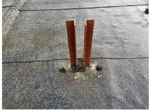
Redundant supports are being removed during the refurbishment works.
