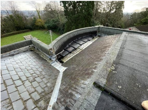
Further overview of the existing roof area.
