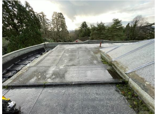
General overview of the existing roof area, opposite side.
