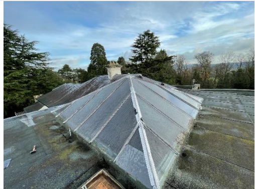
The rooflight is still in use and shall remain in situ. The client has stated that they will carry out the restoration work and bring it back to a suitable condition
