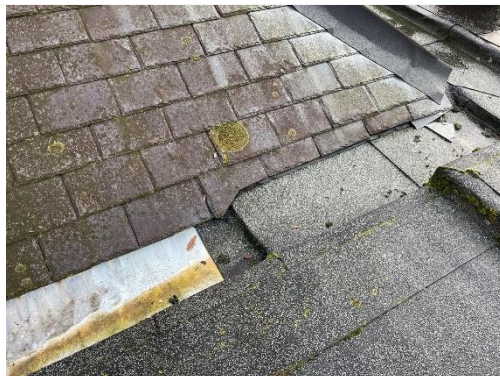
At the pitched roof abutment, the bottom two or three courses of tiles will need to be removed and safely set aside, to allow for the new system to be installed.
