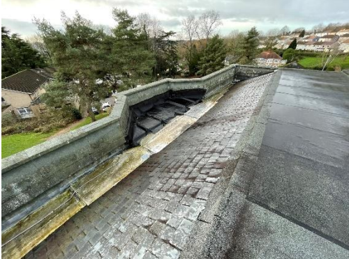
Overview of the existing roof area.
