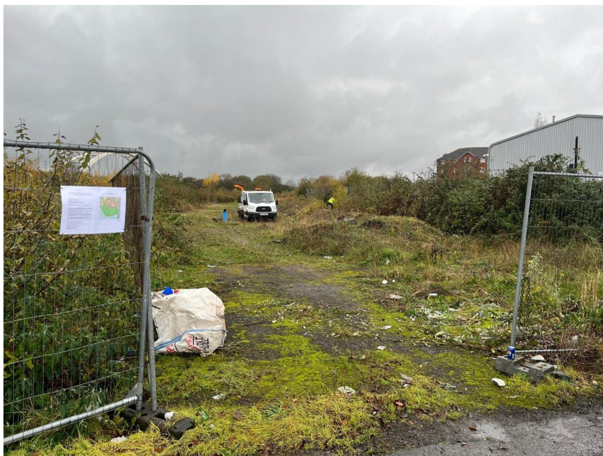
Figure 1: Start on site 18/11/24 – original site conditions
