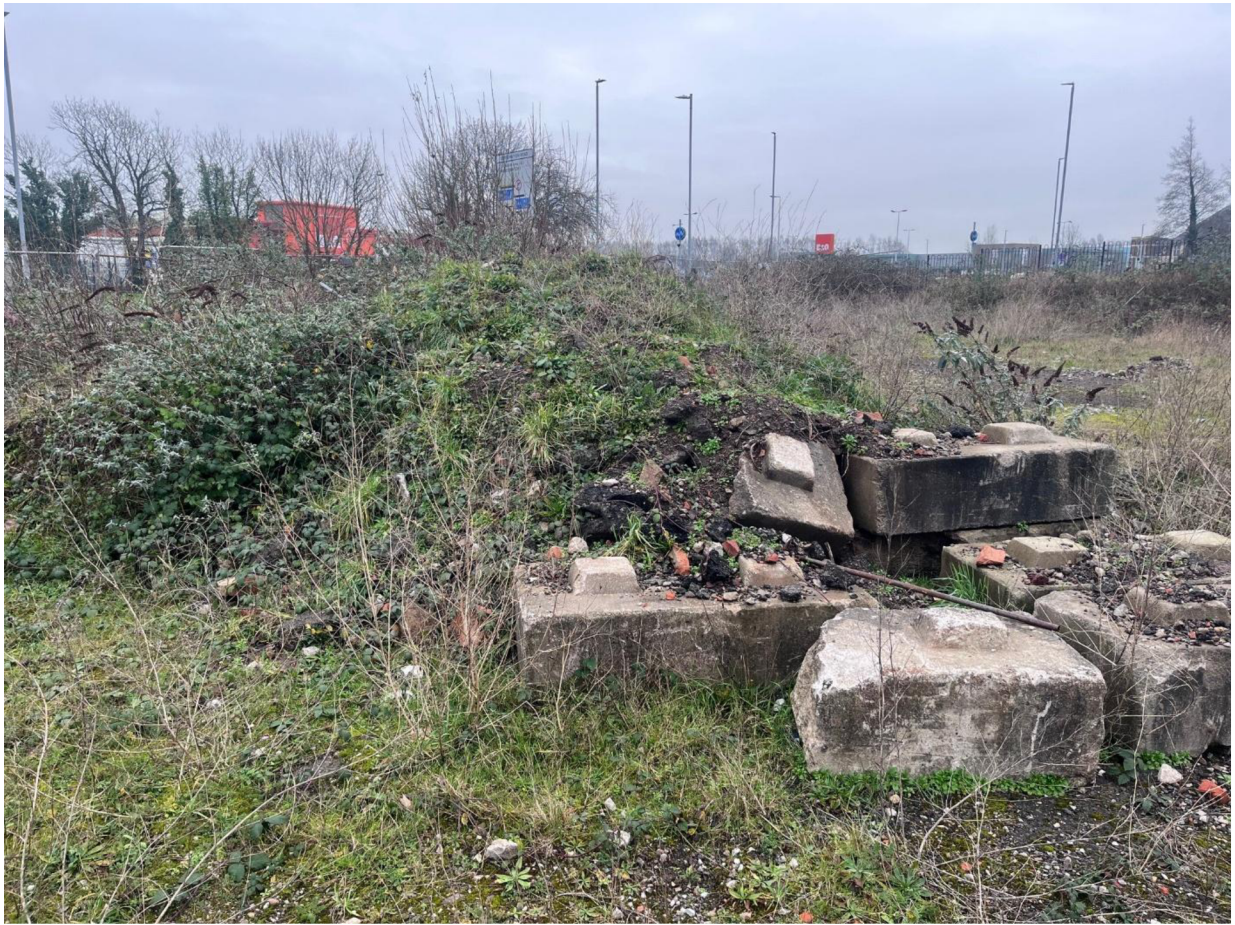
Figure 4: Stantec site visit 26/01/26 - stockpile of material removed from haul road levelling
