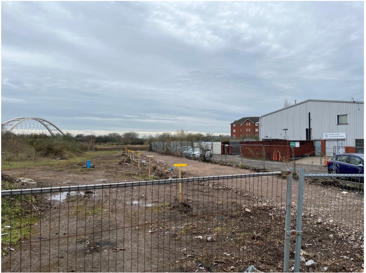
Figure 2: Completion of commencement works and subsequent creation of temporary haul route
