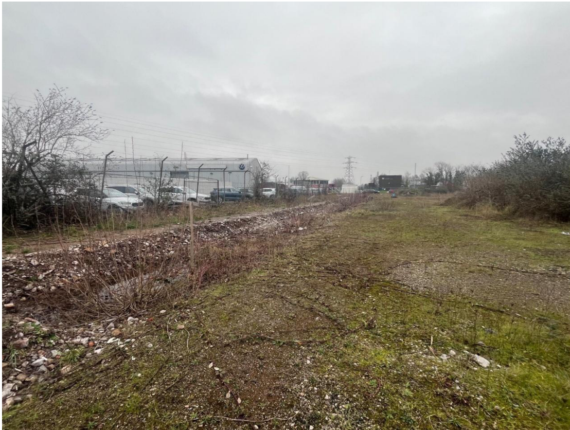
Figure 3: Stantec site visit 26/01/26 - extent of works and haul road
