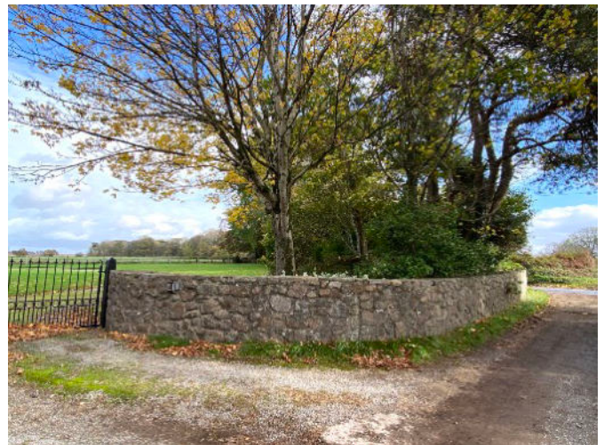
Southern site boundary stone and mortar wall to the east of the entrance gate
