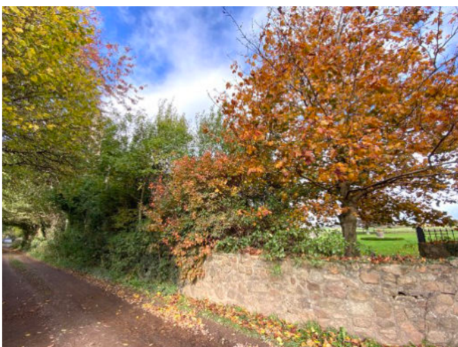
Southern site boundary stone and mortar wall and tree line to the west of the entrance gate
