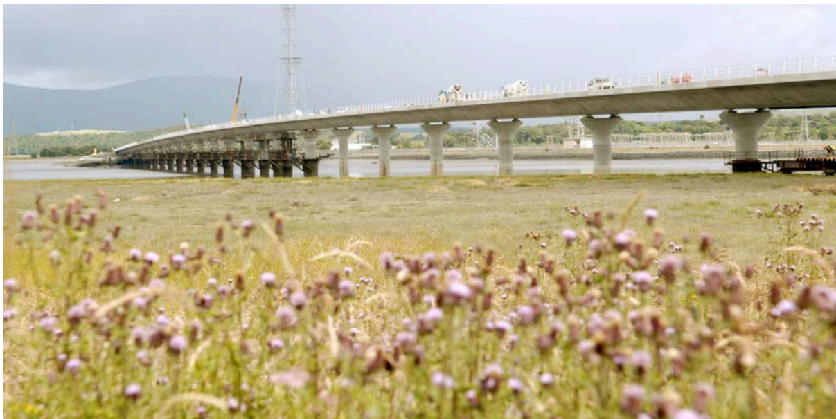
Bridge maintenance (courtesy of SEPA)
