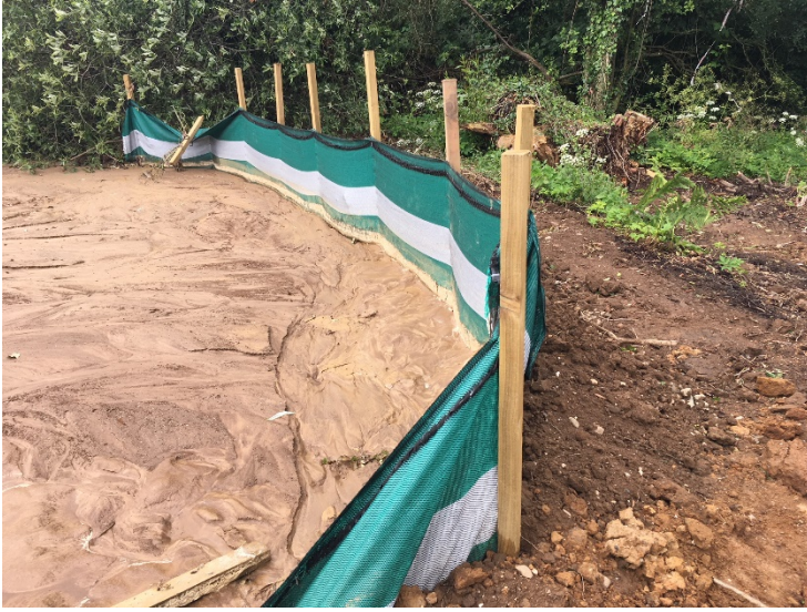
Figure 3: Typical Silt Fencing Set-up
