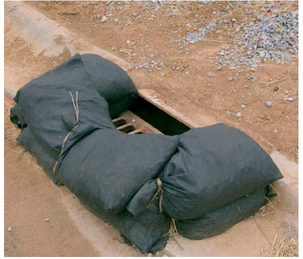
Figure 4: Typical sand-bag set-up to intercept silts before entering drainage systems.
