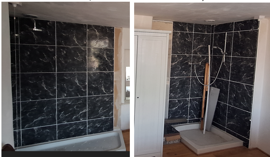
Fig 8 & 9 Partially Completed Bathrooms
