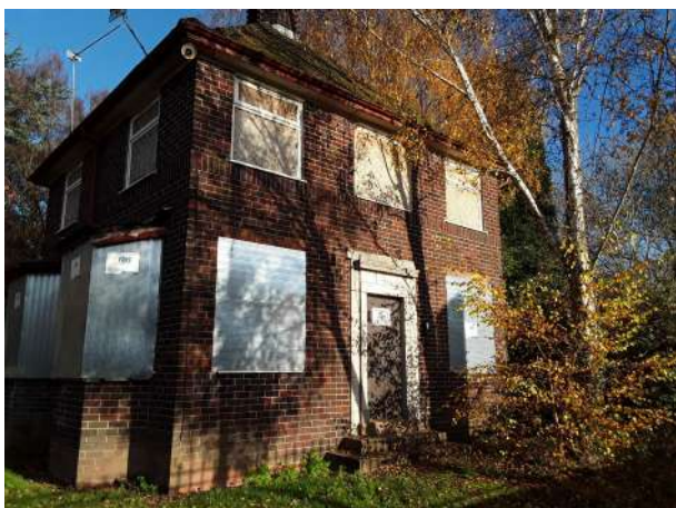
Photograph 13: Building S1 with high bat roost potential.
