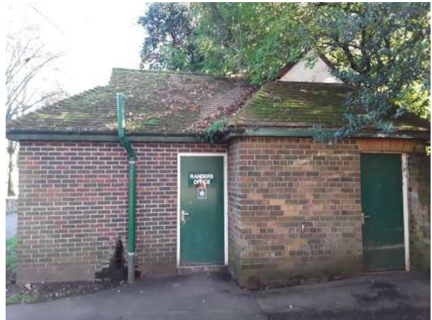
Photograph 20: Building S2 with high bat roost potential
