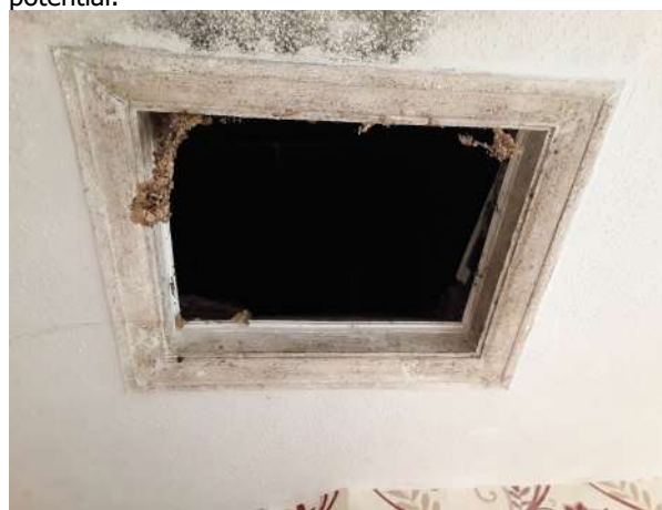
Photograph 16: permanently open loft hatch of building S1 leading into loft space.
