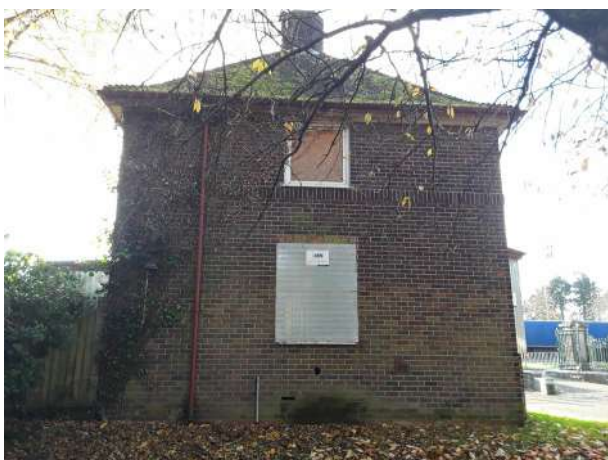
Photograph 15: Building S1 with high bat roost potential.
