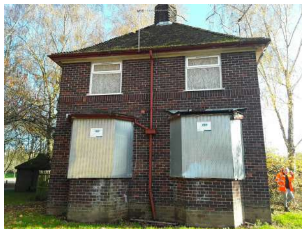
Photograph 14: Building S1 with high bat roost potential.
