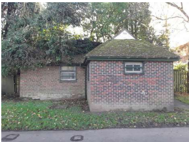
Photograph 17: Building S2 with high bat roost potential.
