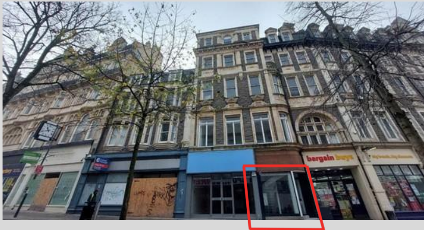
Entrance to the building marked with red lines.
