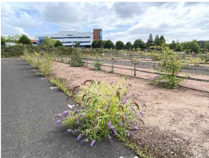
Loose stone hardstanding and vegetation at northern end of former car park, viewing east
