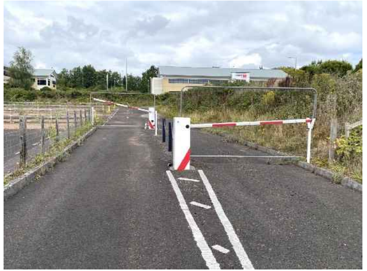
Security gates inside of north east boundary mound, viewing north west
