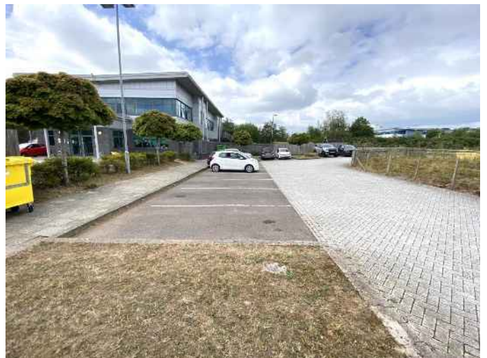
Brick weave and tarmac hardstanding at south end of the site, viewing west
