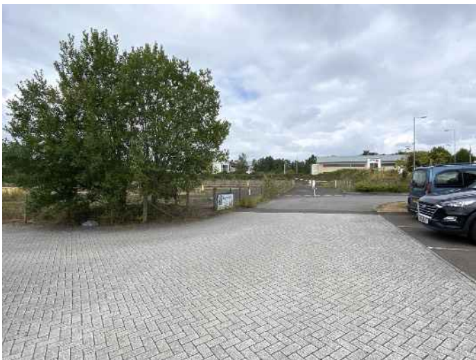
Brick weave hardstanding at south end of the site, viewing north
