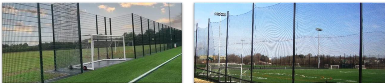
Figure 5 - Twin-Wire Rebound Perimeter Fencing and Ball Stop Netting
