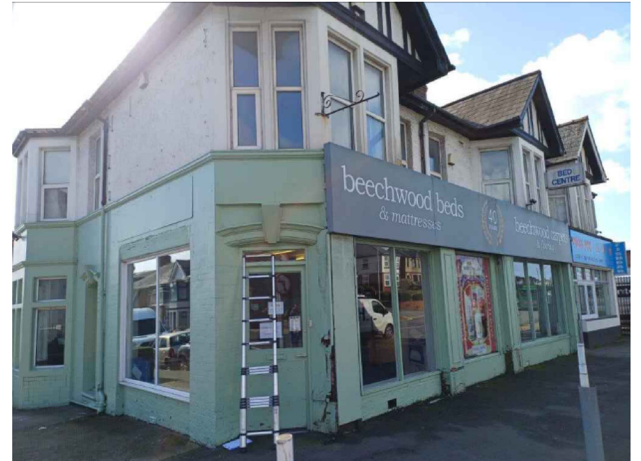
PHOTO OF EXISTING FRONT ELEVATION
