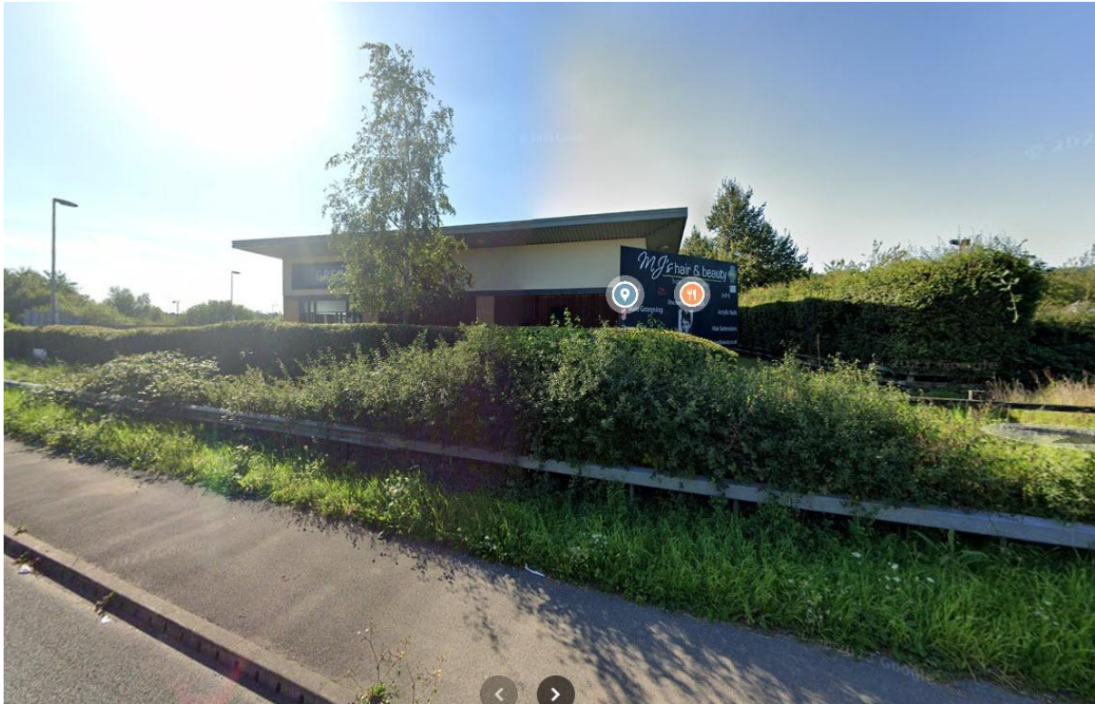
Photograph of Existing MJ's Beauty Sign (to be removed)
