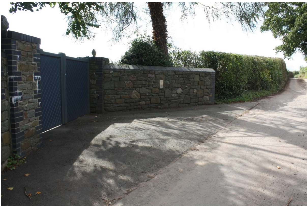
Adjoining access serving The Barn to the South West.
