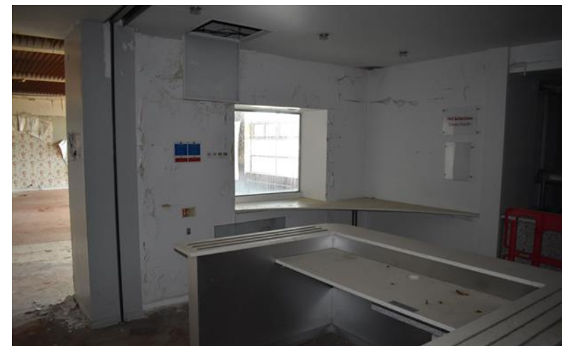
Figure 4.3: : Internal appearance of the extension (top) looking towards stud partition with Resident's Lounge (bottom) looking to surviving original stone walls at the northwest corner of the extension.
