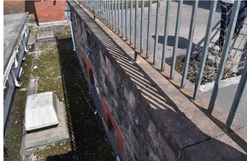
Figure 3.6: Brick dressed windows below the parapet on the northwest facing elevation of the extension.
