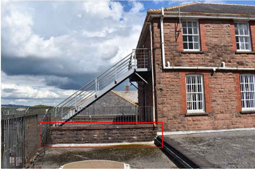
Figure 3.5: (left) Extension parapet (in red) – southwest facing elevation
