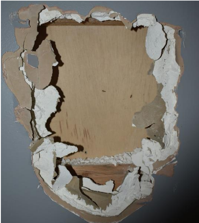
Figure 4.2: view of the construction of the panelled north wall of the Residents Lounge
