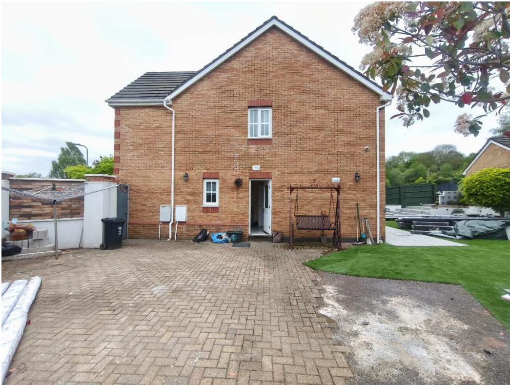
Picture 1: View of South elevation where conservatory is proposed
