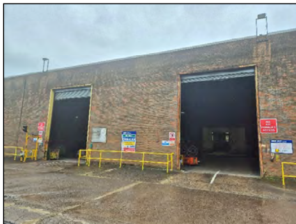
Figure 11 – (NW) Aspect of Shed 6. Open Roller-Shutter Doors and Gaps around Tops of Doors when Closed Offer Potential Access/Egress to Interior for Bats
