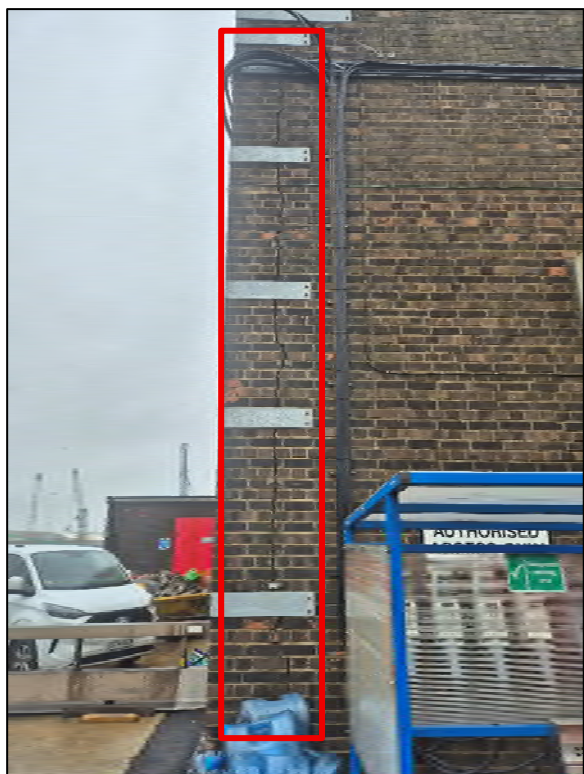
Figure 12 – Crack within Brickwork at (SW) Corner of Shed 6 Exterior Offers Some Limited Roosting Potential for Crevice-Dwelling Bats
