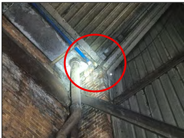
Figure 21 – Detail of Steel Framework and Single-Skin Steel Sheet Cladding Making up Roof of Shed 6. Cladding Observed in Generally Excellent Condition Although a Small Hole was Recorded which May Permit Access/Egress for Bats
