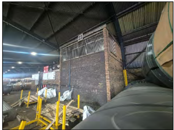
Figure 18 – Additional view of Brick Structure within Shed 6. Brickwork Observed to be in Excellent Condition
