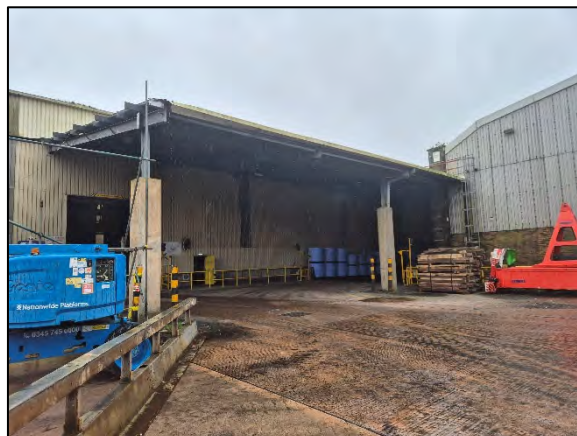
Figure 5 – (NE) Corner of Lean-to, Looking (S)
