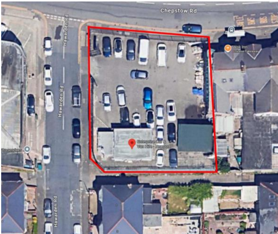
Image 2: Aerial View of the site
