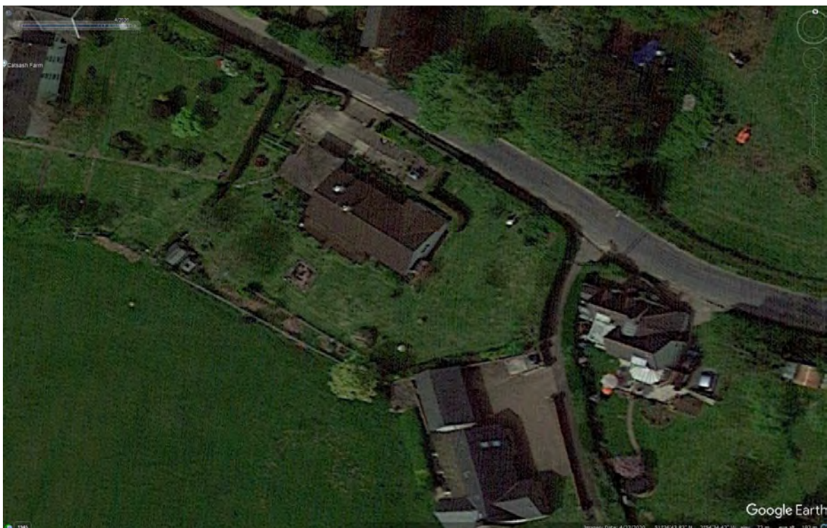
(x) Aerial image of Catsash Bungalow (GoogleEarth, April 2020)
