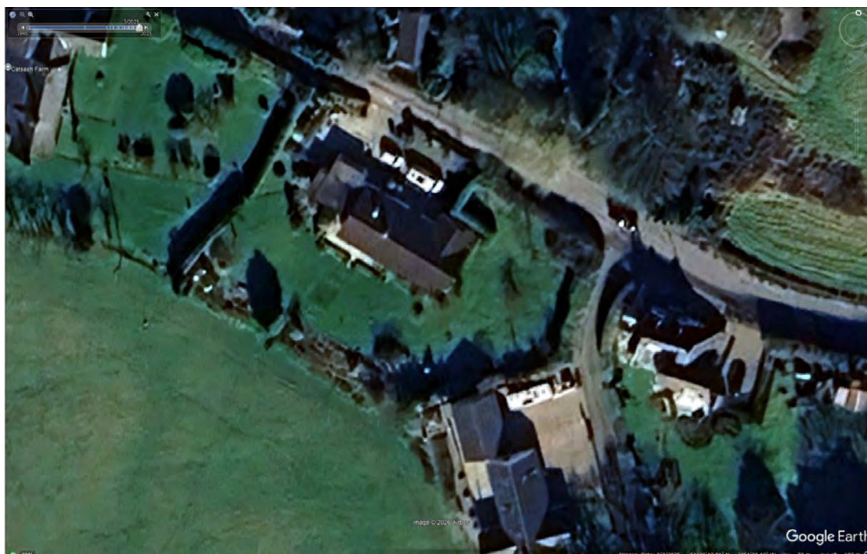
(xii) Aerial image of Catsash Bungalow (GoogleEarth, March 2025)
