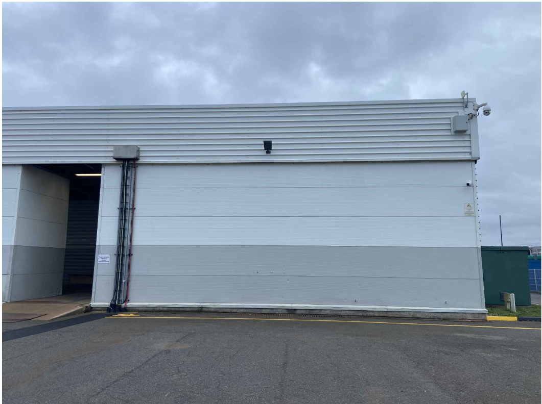
EXTERNAL ELEVATION OF GENERATOR ROOM
