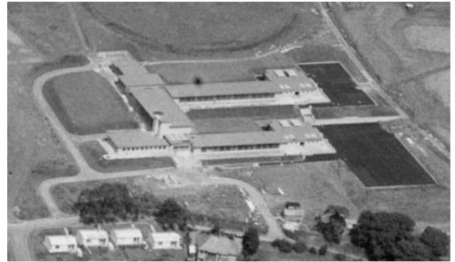
Above (right): 'Britain from Above' aerial image of the school soon after completion (circa early 1950s). Note absence of rooflight in question.
