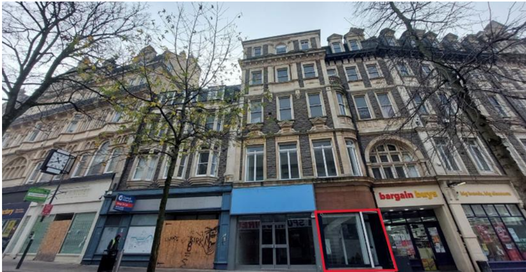
Entrance to the building marked with red lines.
