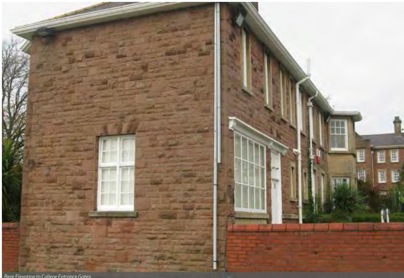
Rear Elevation to College Entrance Gates
