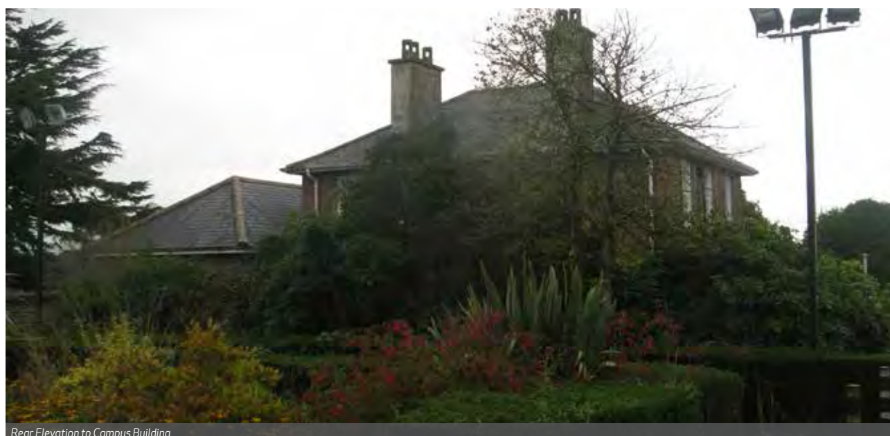
Rear Elevation to Campus Building
