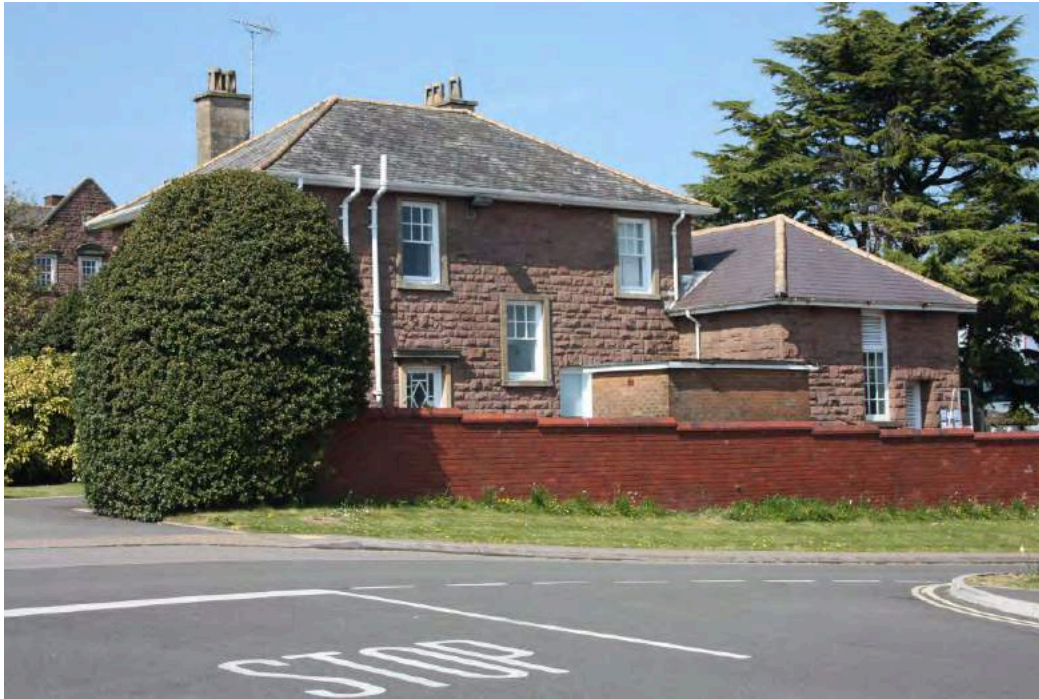
Plate 5: The caretaker's or gardener's lodge
