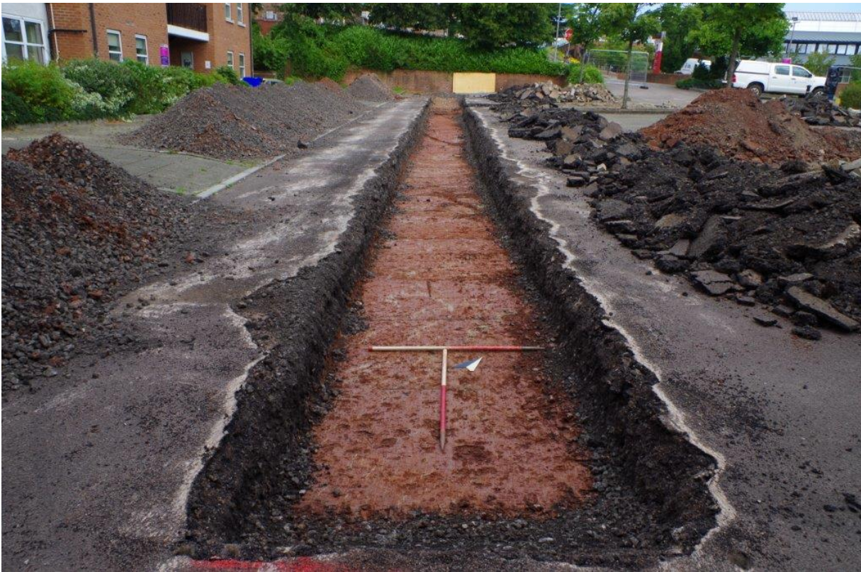
Plate 1 Trench 23, looking north-west (1m scales)
