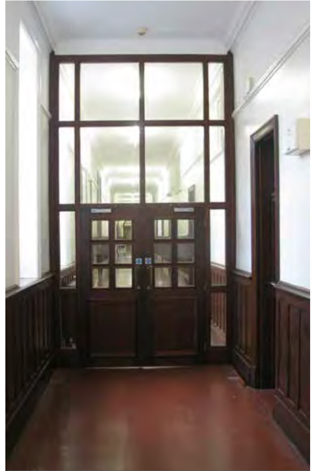
Fire Doors Corridor, Administration Block
