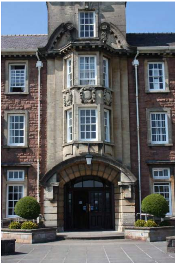
Plate 6: Central frontispiece of the main façade
