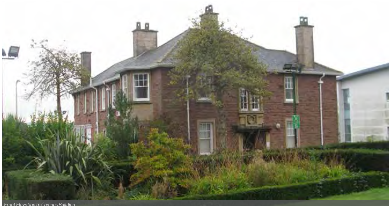
Front Elevation to Campus Building
