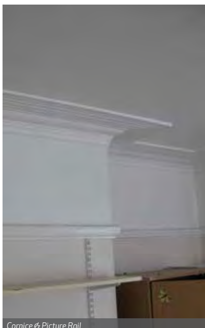
Cornice & Picture Rail
