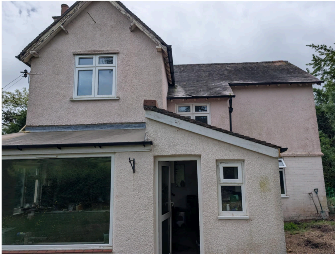
Plate 4-example of sealed eaves
