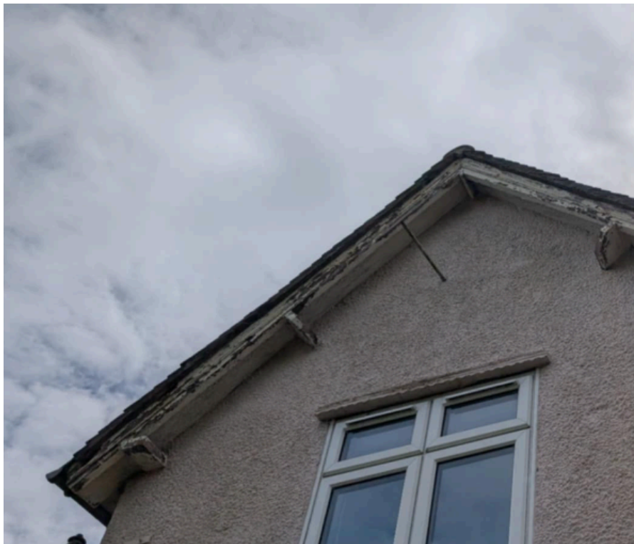
Plate 6- close up of sealed eaves (example)
