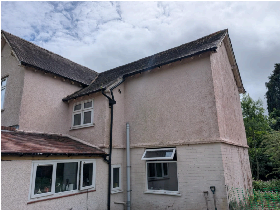
Plate 4-example of sealed eaves
