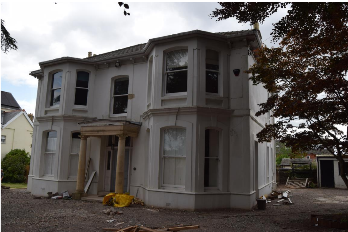
Plate 2: View looking NE towards the front elevation of No. 46 Caerau Road.
