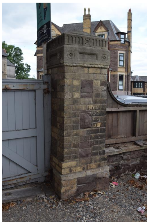
Plate 10: View looking NW, focusing on one of the pier of the N gate to No. 46 Caerau Road.
