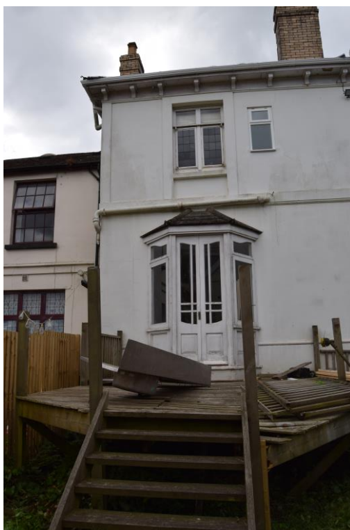
Plate 3: View looking S, towards the N-facing elevation of No. 46 Caerau Road.
