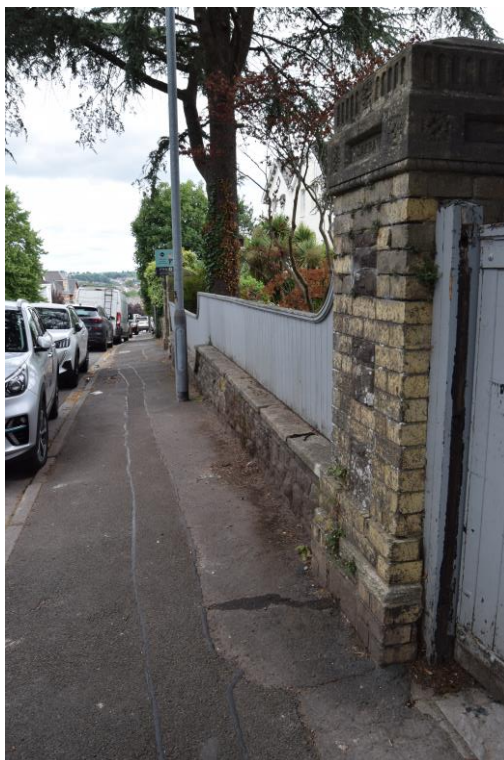
Plate 5: View looking NNE long the front boundary of the site.
