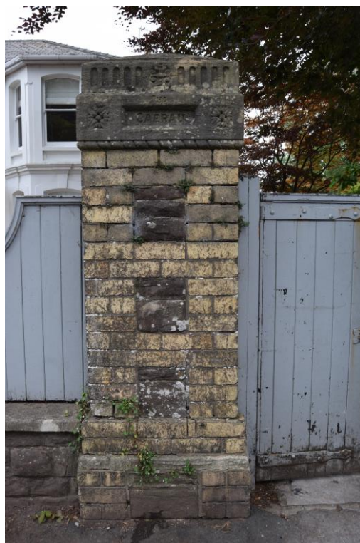
Plate 8: View looking E, showing a closer view of a pier to the S gate.
