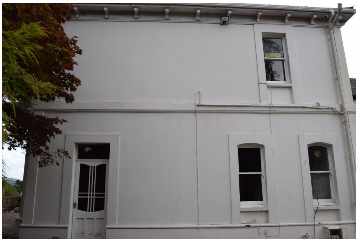
Plate 4: View looking N, towards the S-facing elevation of No. 46 Caerau Road.
