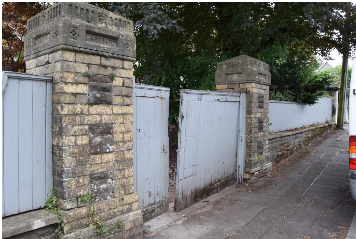
Plate 7: View looking SSE, towards the S gate to No. 46 Caerau Road.
