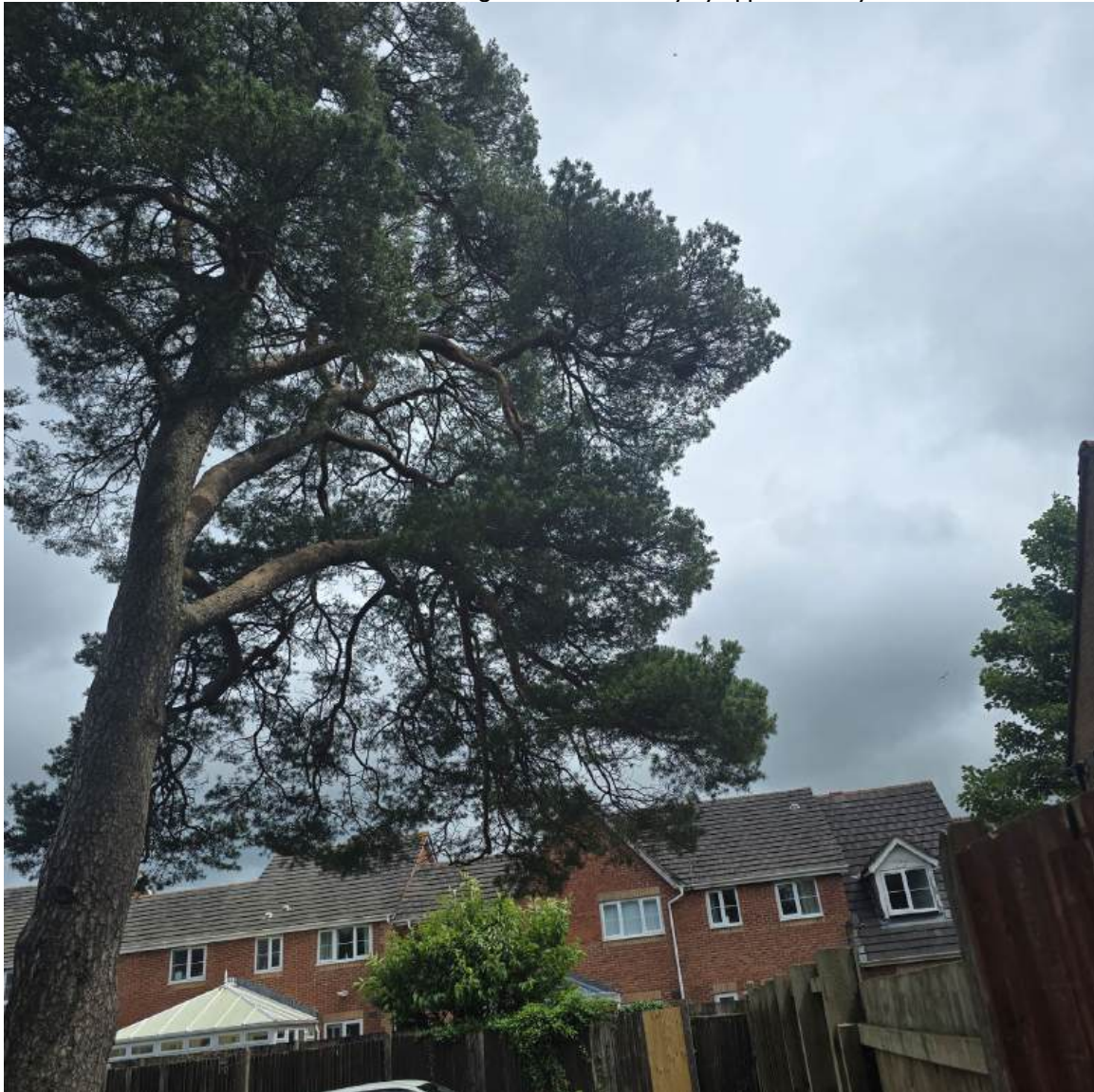
Photo 3: T1 . Crown overhangs the site boundary by approximately 0.2m.
