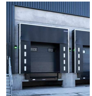
Pre-cast insulated concrete wall with inset overhead sectional doors and dock shelters
