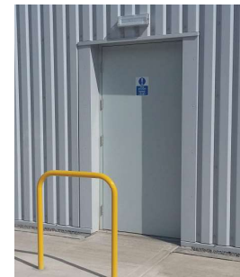
Insulated steel emergency exit/personnel doors
