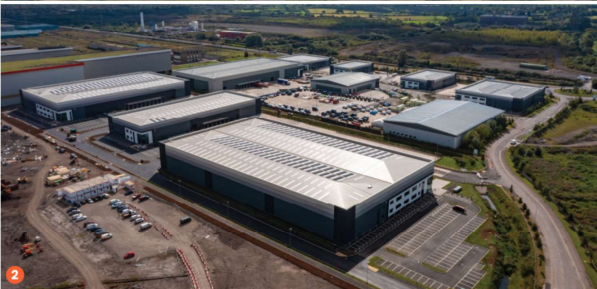
Aerial views showing the Newport Indurent Park
