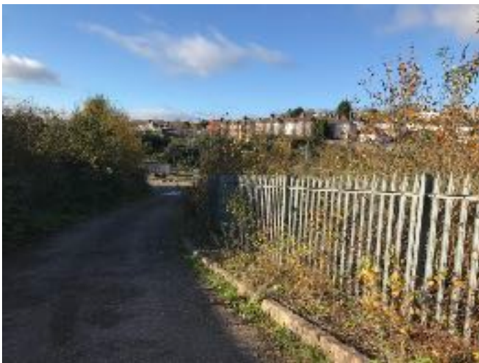
Fig.10 - Palisade fencing along south east boundary
