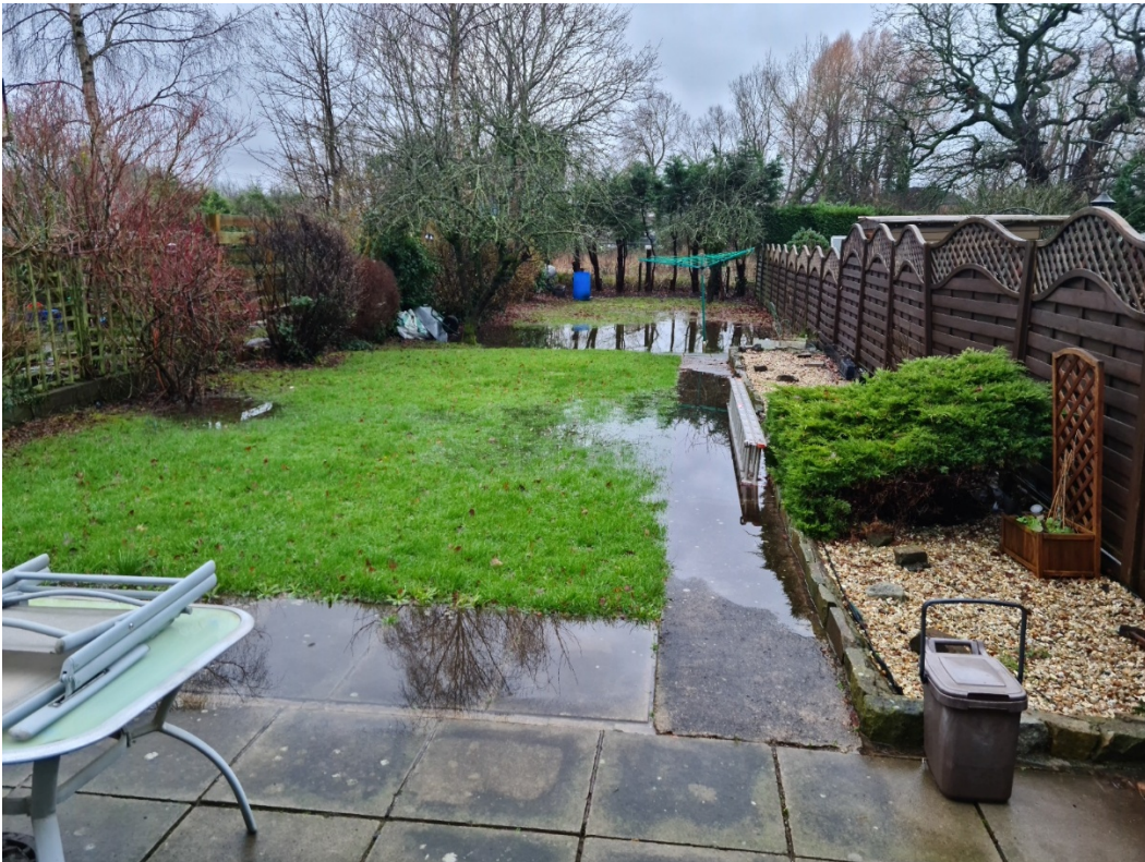
Figure 3 Flooding - garden of 15, Traston Close and perspective of differing levels
