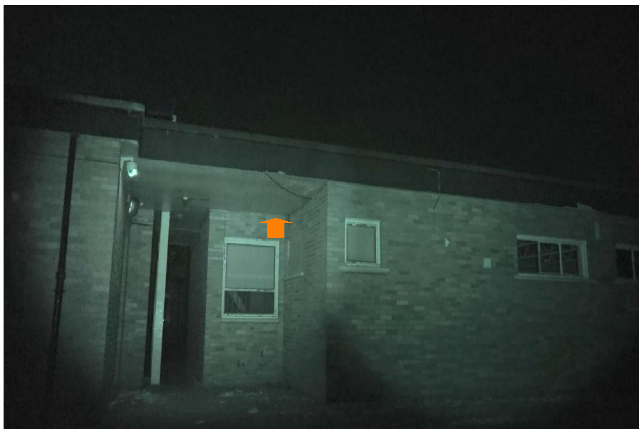
PLATE 1. Building K where evidence of roosting bats was identified
