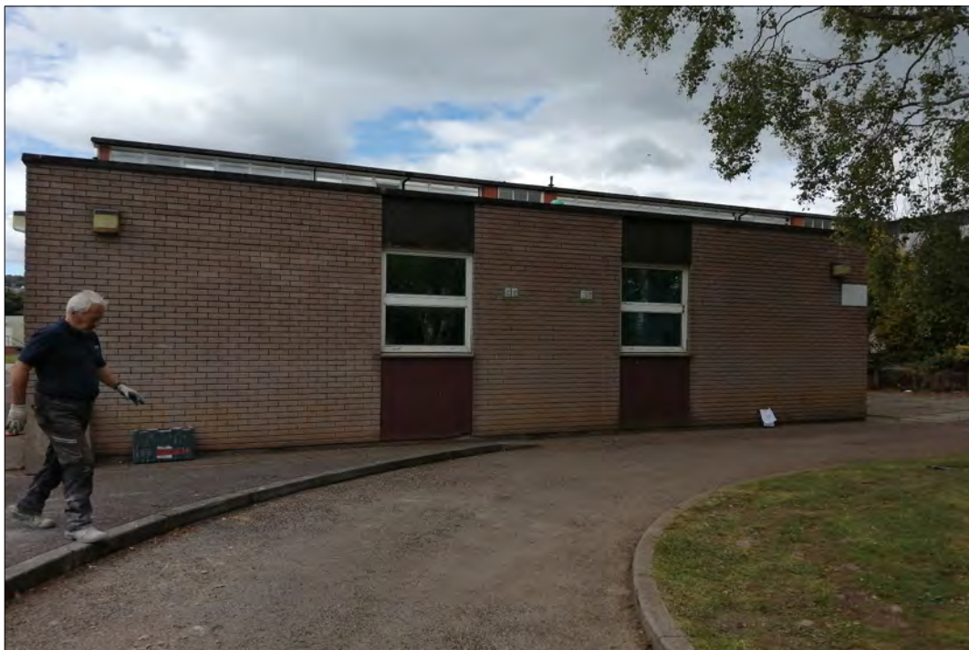
PLATE 16. Building G – WBQ (Target Note 16)
