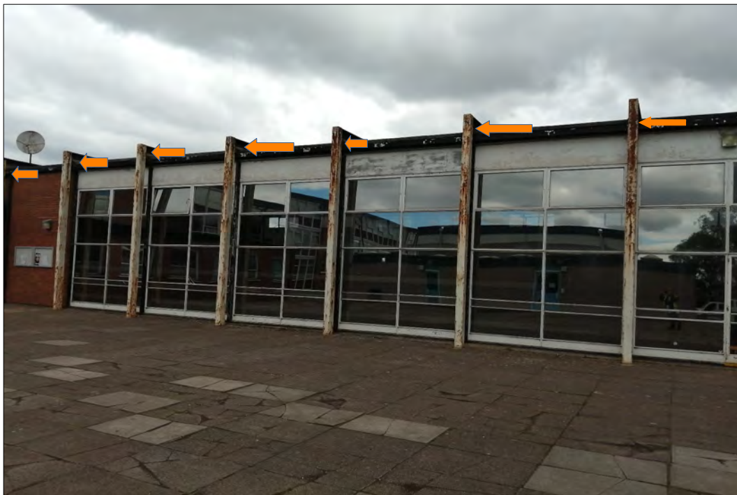
PLATE 8. Building A – Main sports Gym (Target Note 5)
