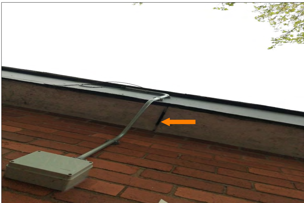
PLATE 5. Building K – Conference building rear showing gap in soffit box underside (Target Note 3)
