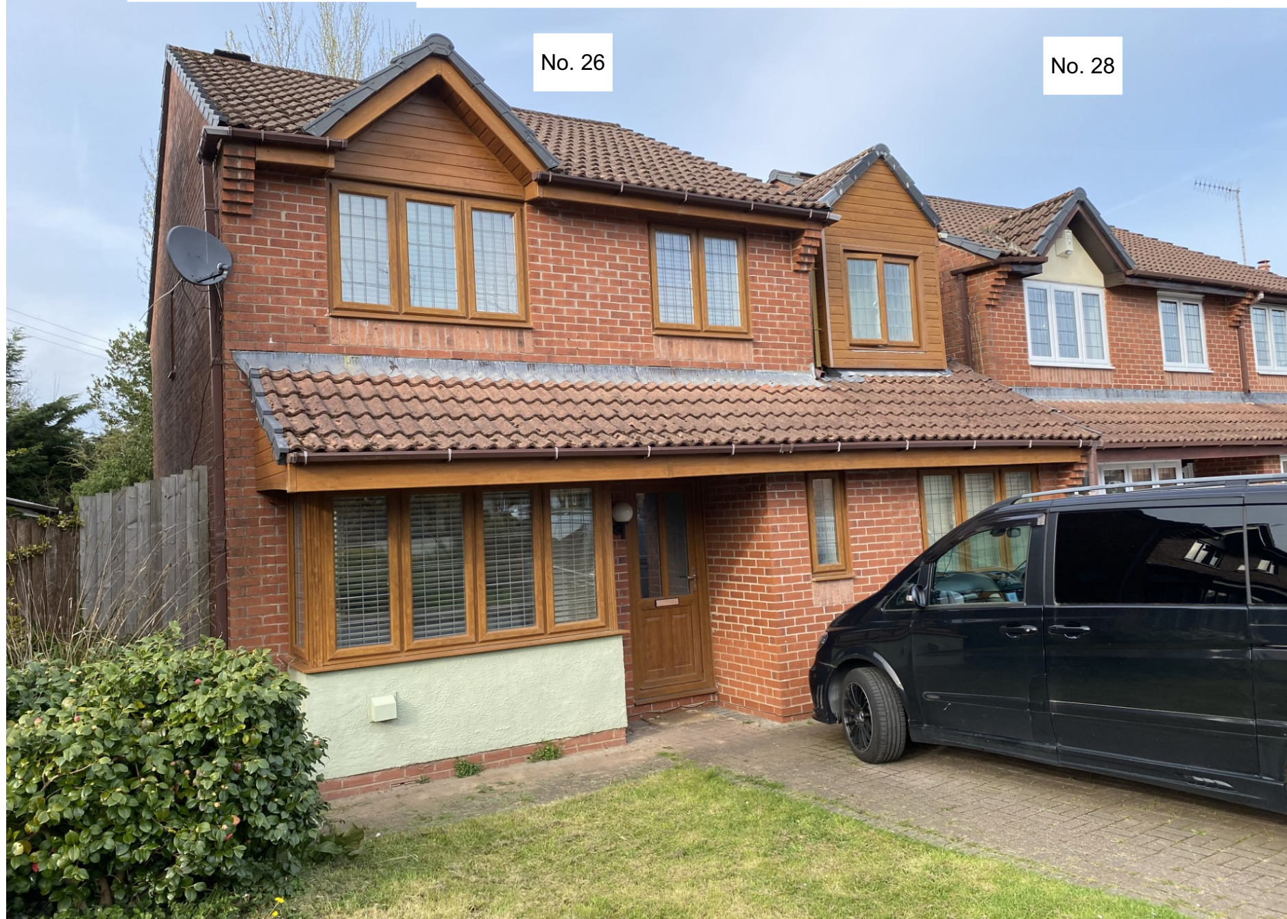
556-2 EXISTING FRONT ELEVATION PHOTOGRAPH - 26 HARLECH DRIVE, RHIWDERIN, NEWPORT NP10 8QS
