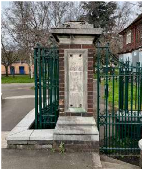
Left: The south and west elevations of the Lodge contain the buildings most ornamental features (much of which remain, though in increasingly poor condition). The adjacent original entrance to the Parks is framed by decorative brick and Portland stone gate-piers, its urban character being further enhanced by the ornamental metal gates and railings.
