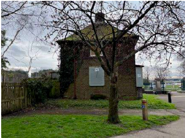
Below: The north elevation of the Lodge, of limited architectural quality.
