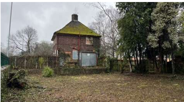
Right A view of the Rangers original garden, looking west. To the south, an ornamental metal fence above a low stone wall separates this garden from the adjacent road. To the north, the Park screened by the existing Outbuilding, flanking brickwork walls, dilapidated timber fencing and mature trees.
