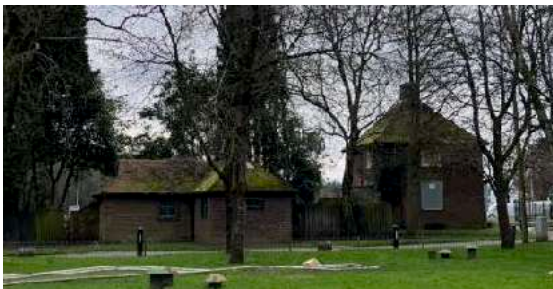
The original Park Rangers Cottage, now known as the Lodge. It's north elevation is visible on the right of this picture, the contemporaneous Outbuilding to its left.
