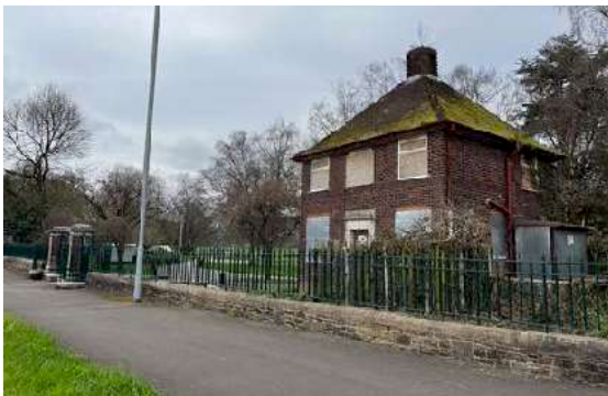
The Lodge's south elevation. Of some architectural quality (the missing original windows notwithstanding), this facade faces the adjacent main road (the A48). The gate piers are visible on the left, these and the Lodge simultaneously constructed to mark the original creation of the 'Tredegar Park Recreation Ground'.
