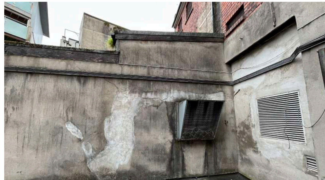
Dilapidated rear facade – significant material decay, defined by weathered concrete, crumbling render, boarded and infilled window apertures. Ad-hoc additions and modifications for plant equipment.
