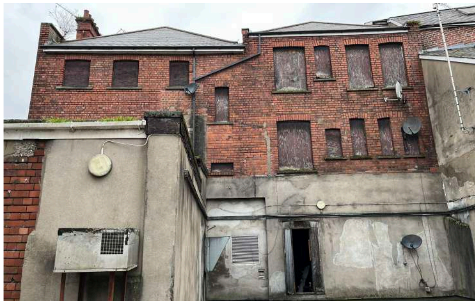
Dilapidated rear facade – significant material decay, defined by weathered concrete, crumbling render, boarded and infilled window apertures. Ad-hoc additions and modifications for plant equipment.
