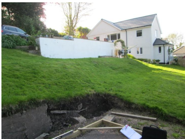
Photo looking north west toward 1 Rising Sun Gardens
