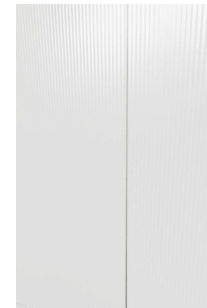
Vertically laid colorcoat Prisma microrib cladding
