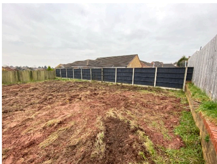
Western boundary vertical wood lap fence with concrete posts and gravel boards, viewing west
