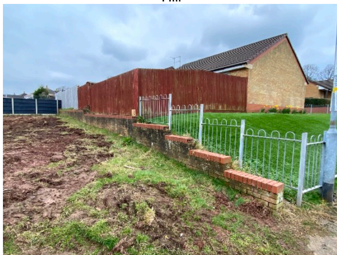
Northern boundary low brick wall and vertical wood lap fence above, viewing west
