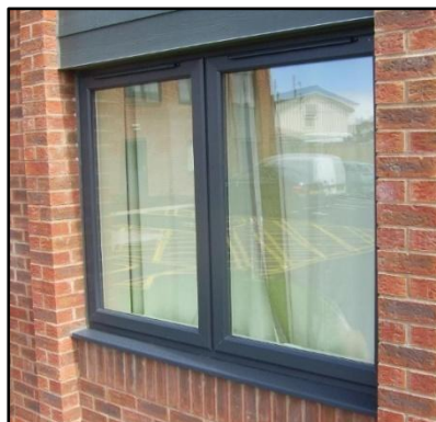
Windows – UPVC windows in RAL Colour 7016
