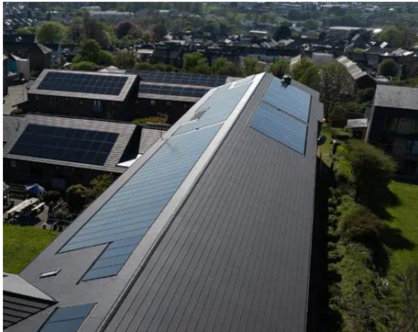
Roofing Material – Marley Edgemere Interlocking Concrete Slate Tile
