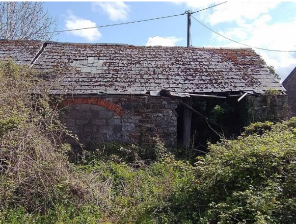
Figure 2 – Southern section of Barn 5 (B5)
