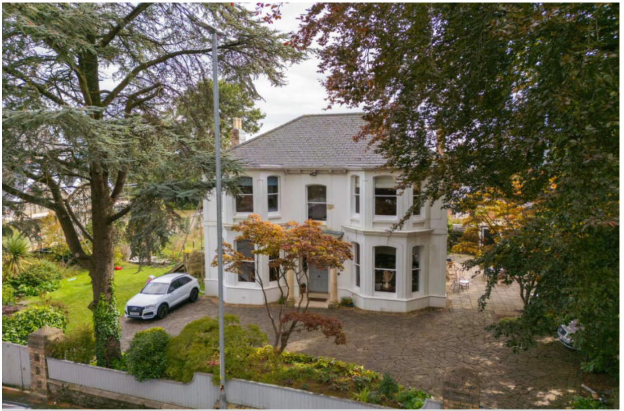
Figure 1 - Arrangement of garden to 46 Caerau Road prior to works taking place.
