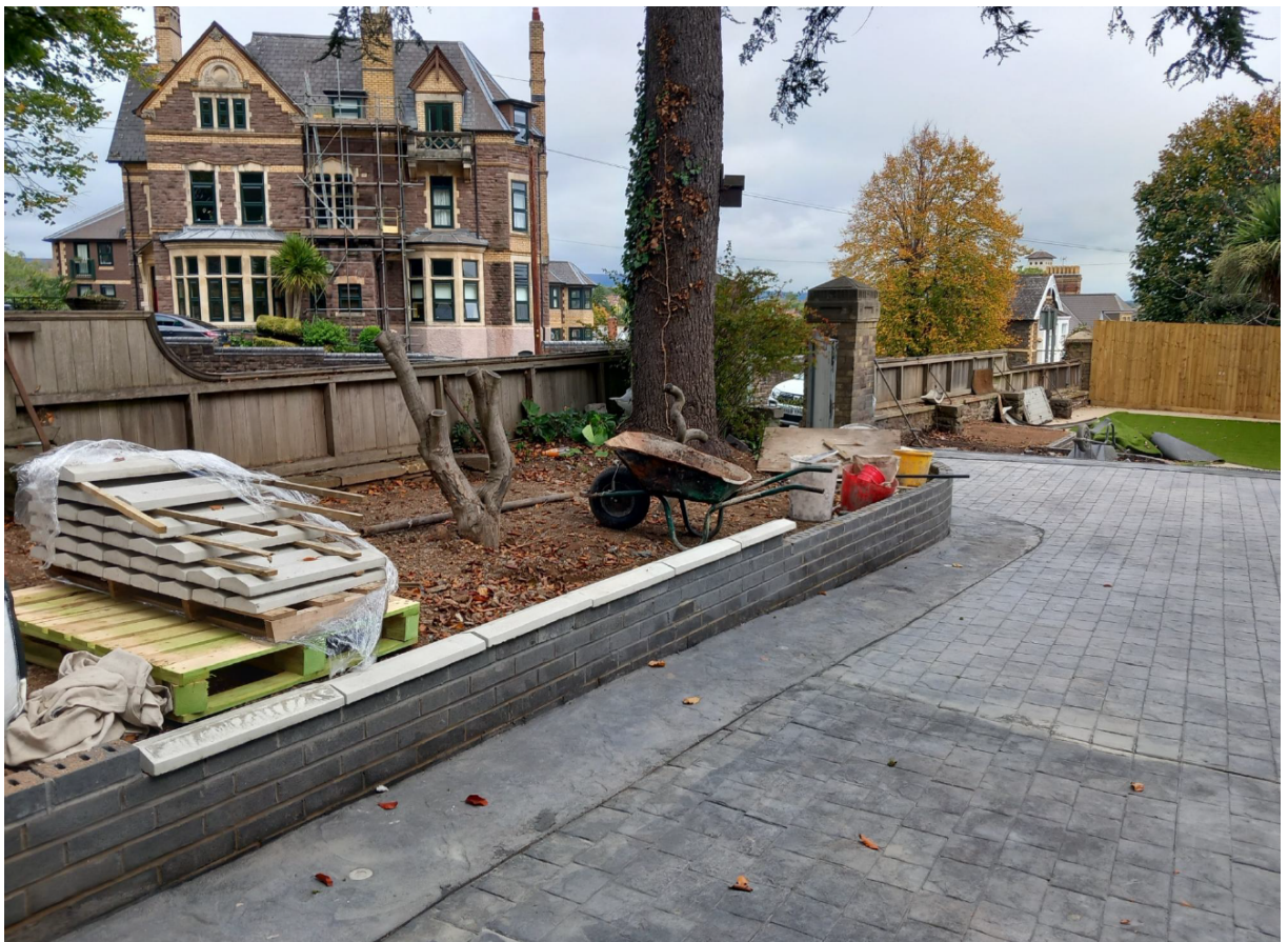
Figure 2 - Existing Hardstanding to 46 Caerau Road - Undertaken without planning permission.
