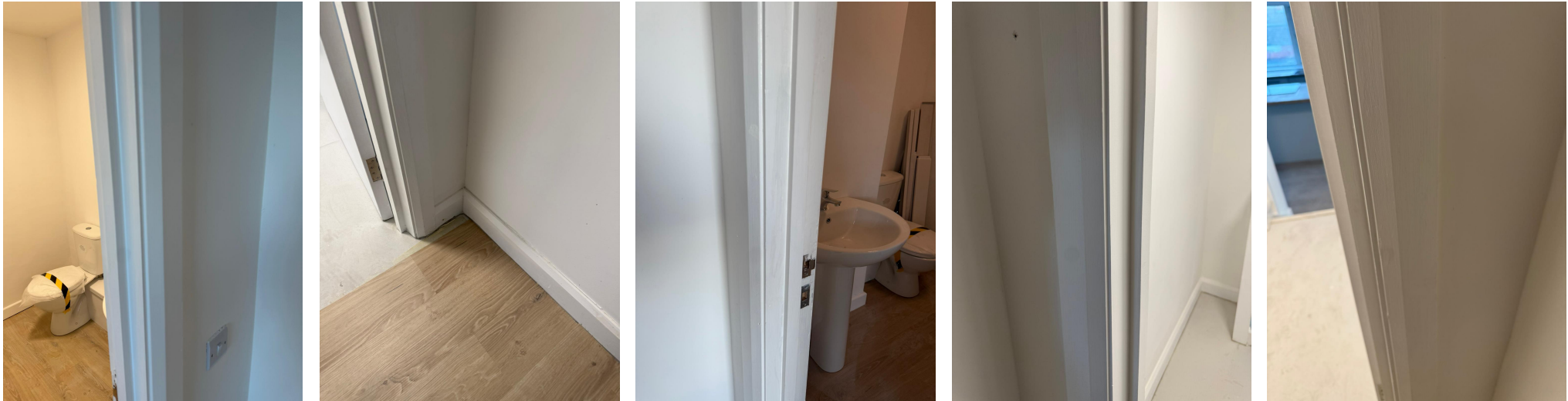
RECORD PHOTOGRAPHS OF EXISTING & REPLACEMENT SKIRTINGS AND DOOR TRIMS (note: existing timberwork replaced only where damaged or layouts amended)
