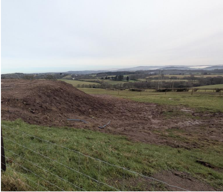
Figure 5(a), Image of bank from yard (Acorus Rural Property Services Ltd, 2025)
