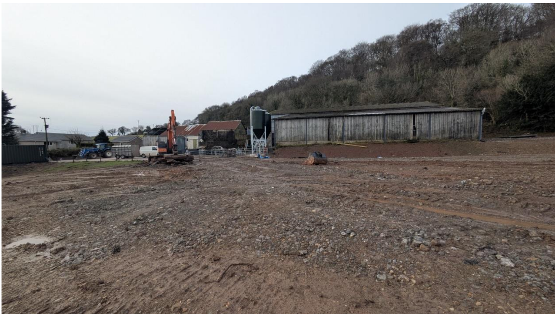
Figure 5(b), Image of bank from levelled area looking west towards the farm complex and woodland (Acorus Rural Property Services Ltd, 2025)
