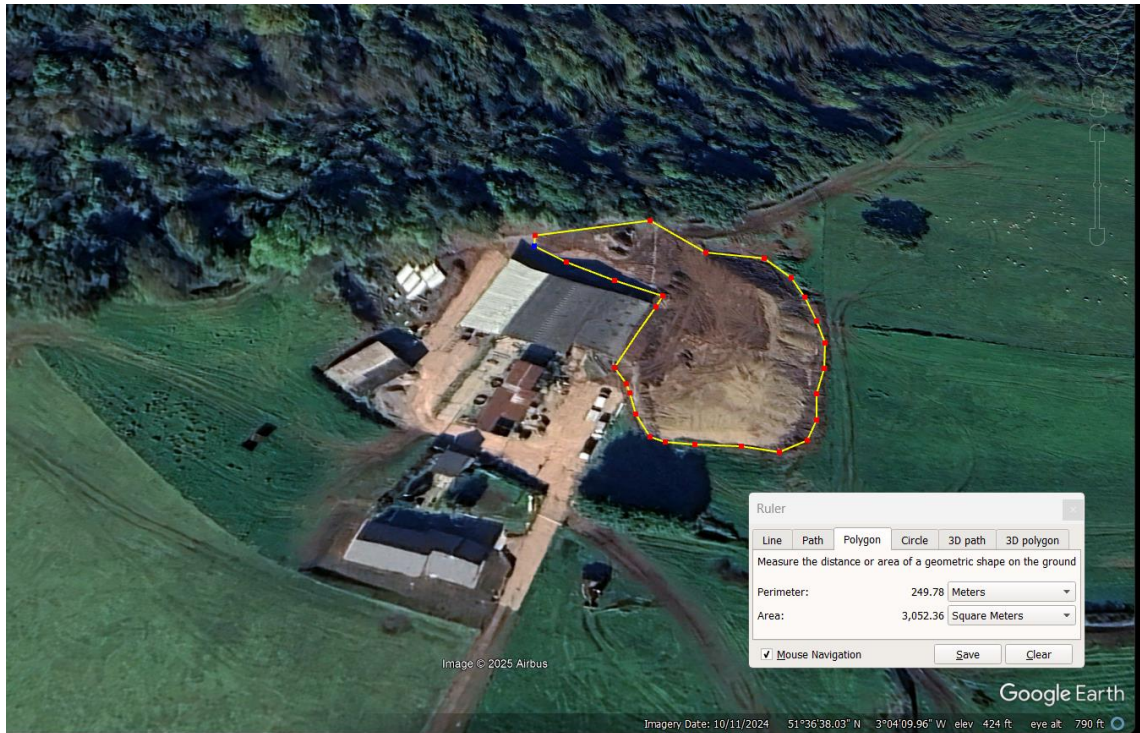
Figure 8, Aerial image showing earth works for ground levelling at Lower Wenallt Farm (Google Earth, June 2025)
