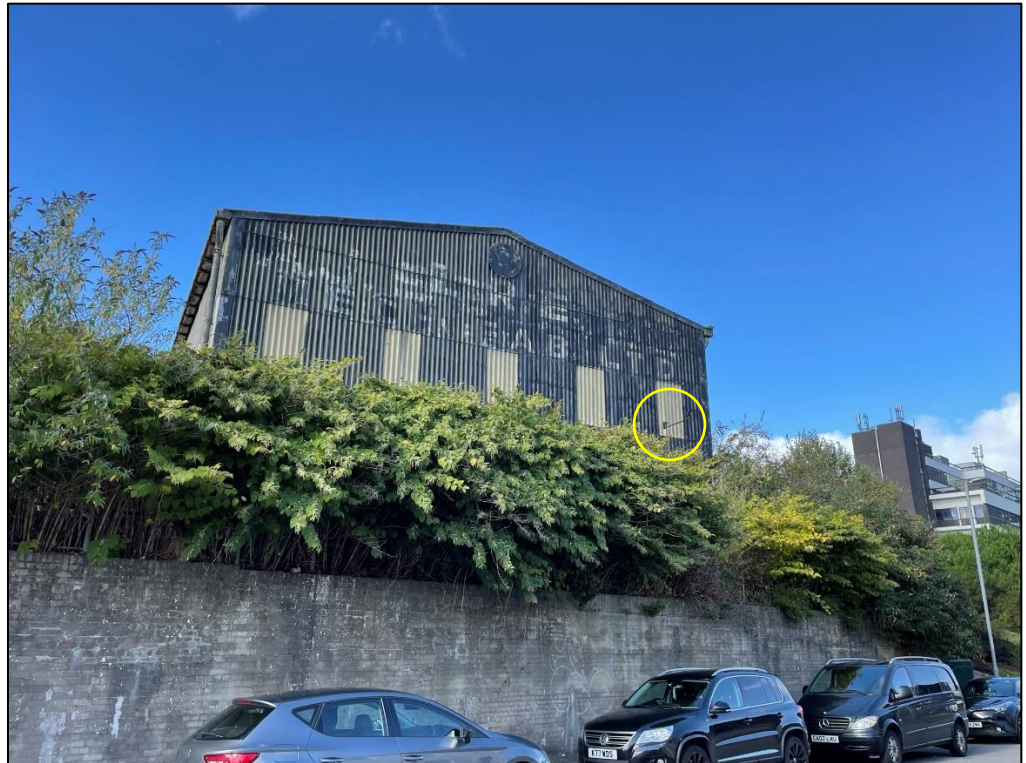
Figure 3 – View of Survey Equipment (Factory Road)
