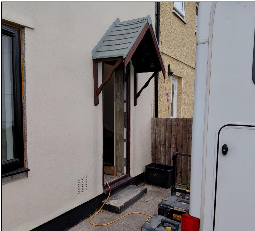
Figure 5: The proposed location of the front porch, facing NE
