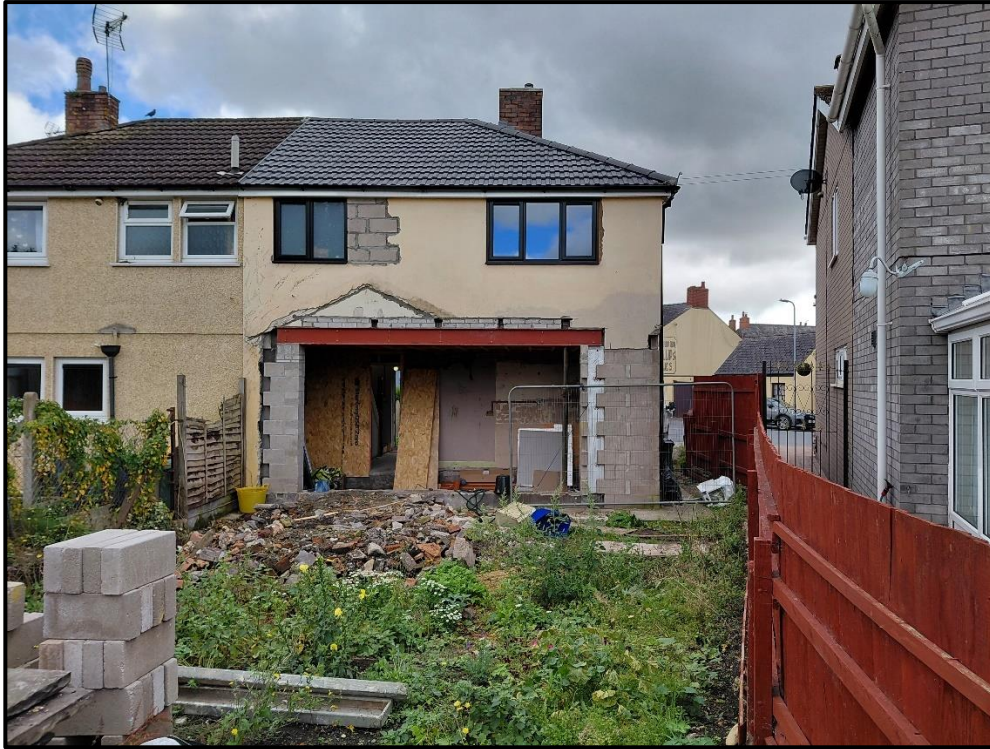
Figure 2: The rear (north-west) elevation of 11 Vine Cottages following demolition of the conservatory, facing SE
