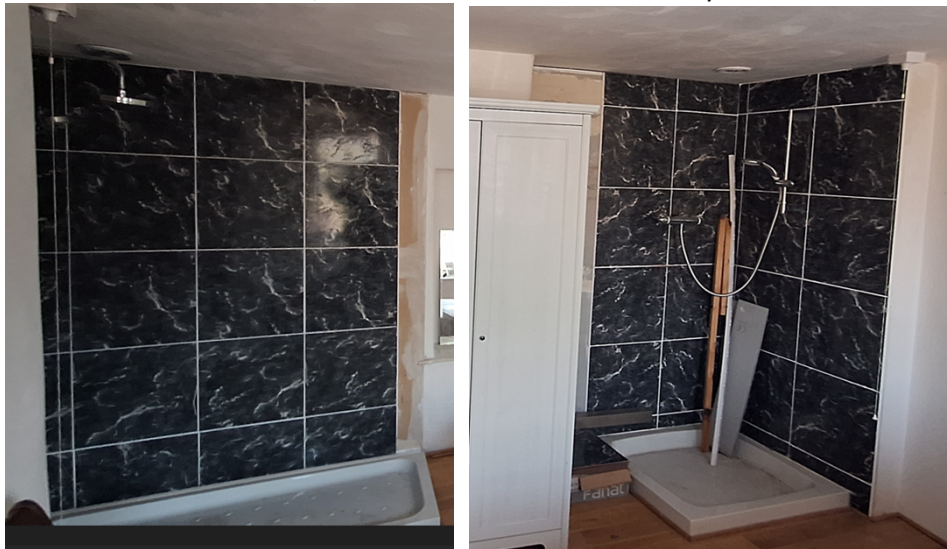
Fig 8 & 9 Partially Completed Bathrooms
