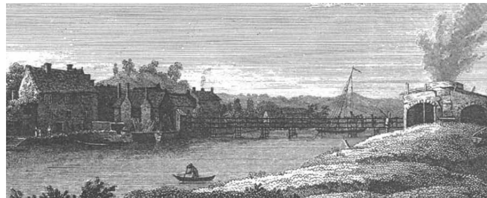
Caerleon Bridge in 1801, illustration by Richard Colt Hoare from William Coxe's Historical Tour In Monmouthshire (source: 'caerleon.net')
