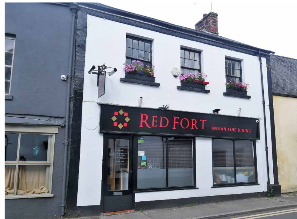
O - 2 Cross Street, June 2021 (source: 'britishlistedbuildings.co.uk')
