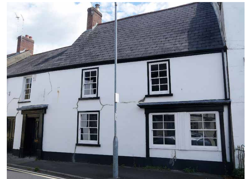
S - 20 & 21 Cross Street, July 2021 (source: 'britishlistedbuildings.co.uk')
