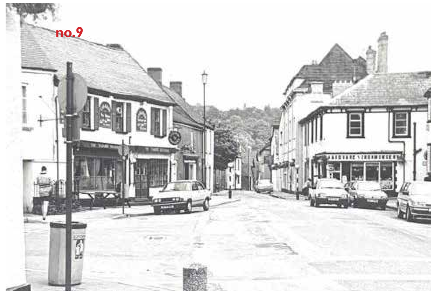
1992 view towards 9 High Street (source: 'southwalesargus')
