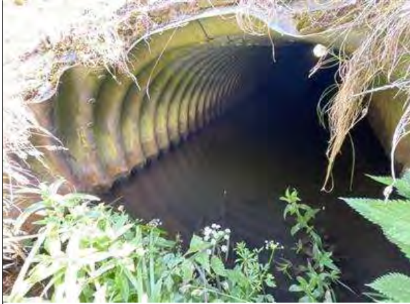
Photograph 7: Culvert under Road to Nature in August 2025
