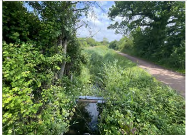
Photograph 16: Percoed Reen at the start of Percoed Lane in June 2025
