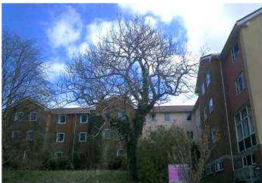
Photograph 18e. Tree 100 – Location of tree with protection afforded by three storey high buildings.
